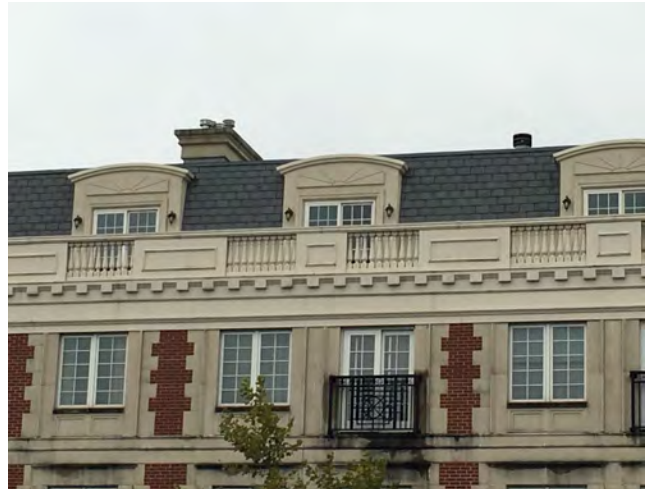
An example of a mansard roof with faux slate shingles
